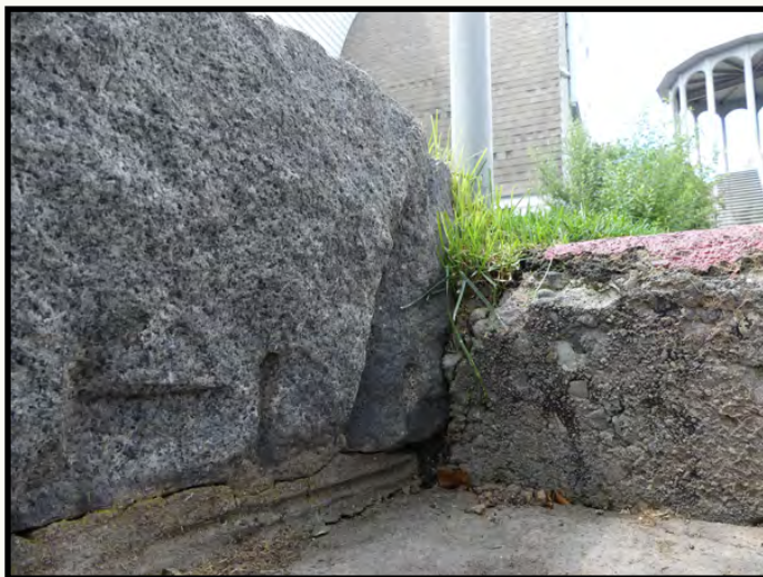
(Above) More evidence on McGlashan retaining wall of Plug and Feather; again note Rocking Stone Tower is in the top right corner
