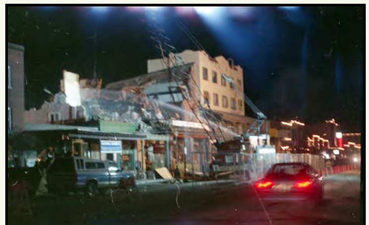
(Above) Masonic Lodge after 1993 Propane Explosion; COR2344
