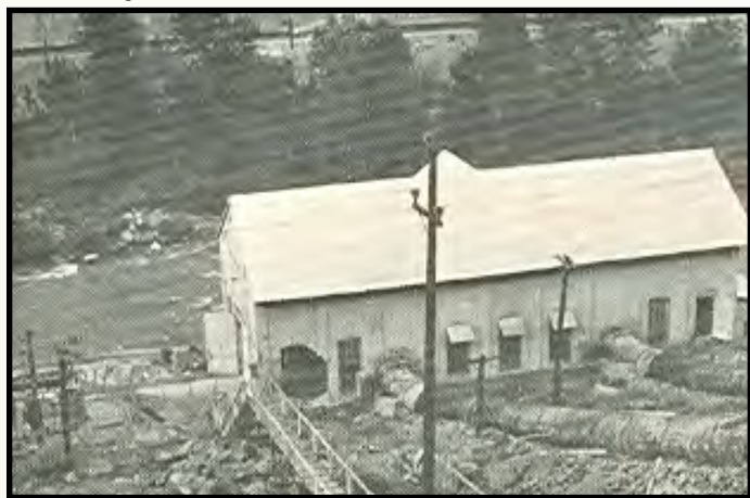
Farad 1966 Quake Damage; photo courtesy Truckee Donner Historical Society
