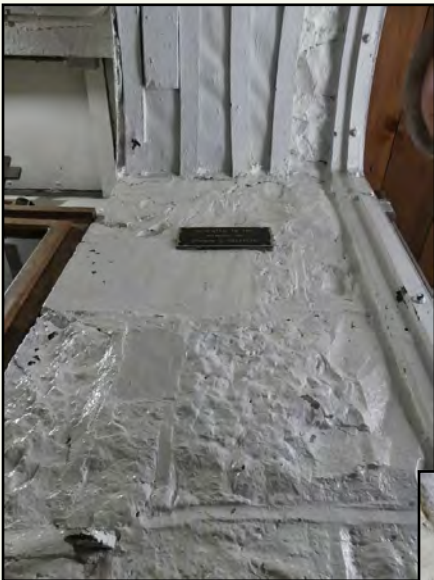
(Above) Note the width of this entrance door
