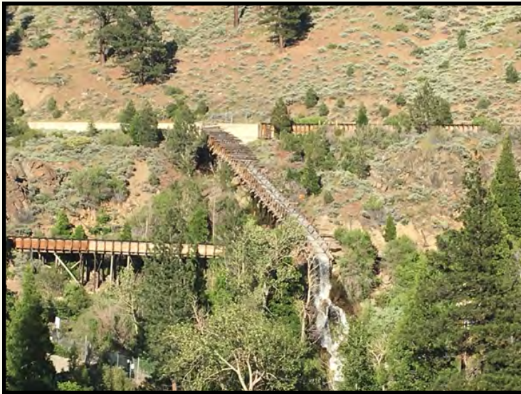
(Above) Spillway off the flume. Photo Courtesy of Kristen Sproat Colley, June 4, 2018.
