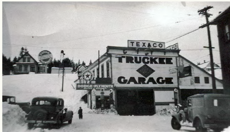
Figure 2 - Truckee Garage would have been where intersection of Donner Pass Road and Spring Street is today; this is where the four buried fuel tanks were discovered
