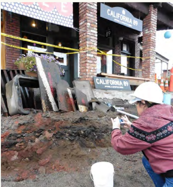
Figure 4 - evidence of fire at the site of the former Sierra Tavern; note the charred wood and evidence of degrading brick; discovered during excavation and work for the Brickelltown Streetscape Project
